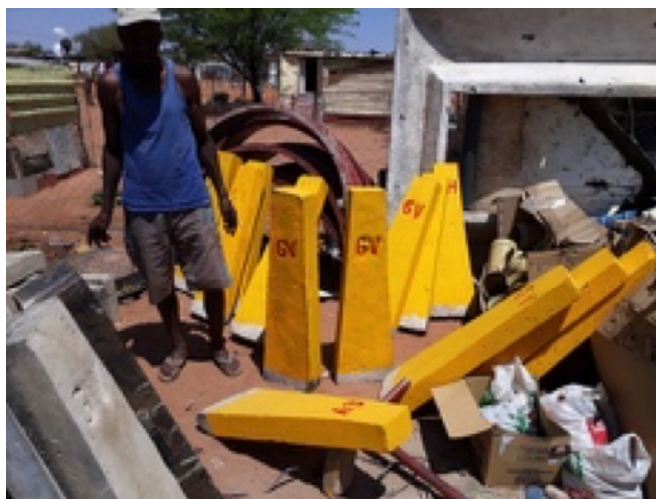
Construction of concrete signs for gate valves and fire hydrants is also done by SDFN/NHAG
